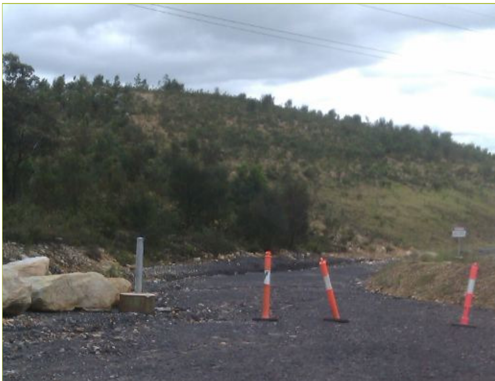
Figure 2.5: Rehabilitation area at West Cliff Colliery
