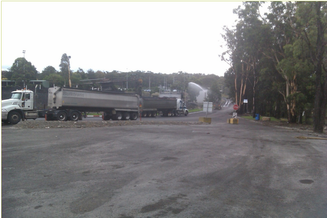
Figure 2.4: Water sprays operating on the stockpile at Appin East
