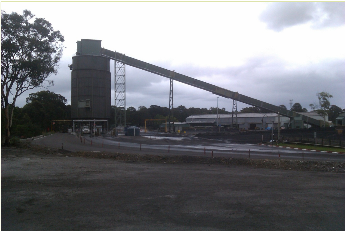
Figure 2.3: Covered conveyor at Appin East Colliery
