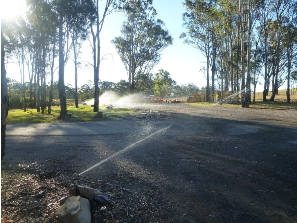
Figure 3.6 Road Sprays on the unsealed road at Appin West
