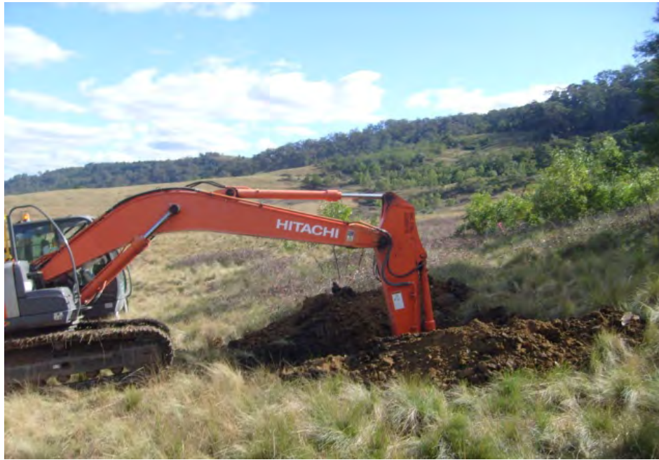
Deep Test Pit In Colluvium Soils Near Toe Of Landslide
