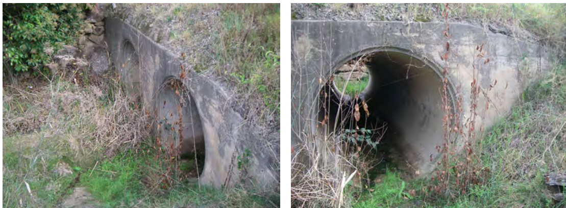
Fig. 6.34 Photographs of Culverts MR-A9-C05 (Left) and MR-A9-C08 (Right)
