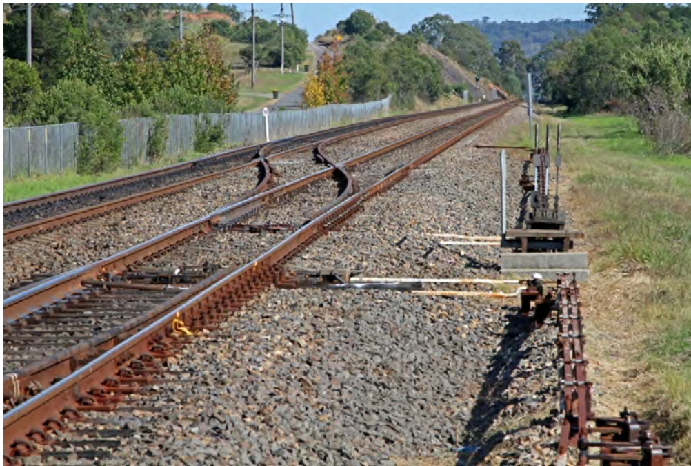
Photograph courtesy Pidgeon Civil Engineering
