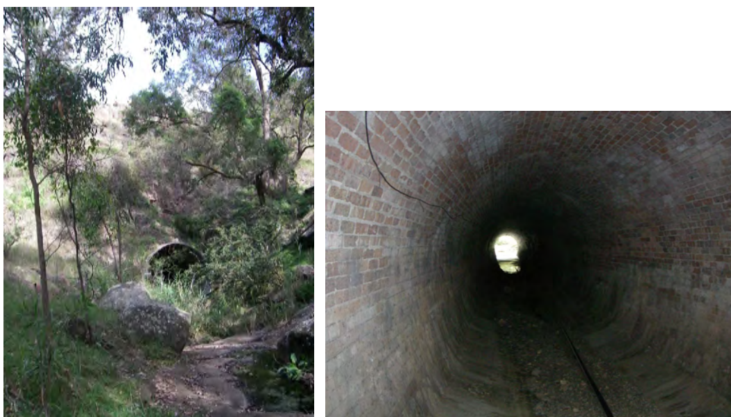
Fig. 6.4 Photographs of Railway Culvert at 75.855 km
