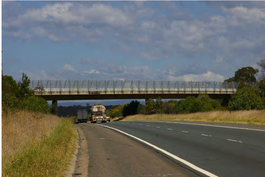
Fig. 6.32 Moreton Park Road Bridge (South)
