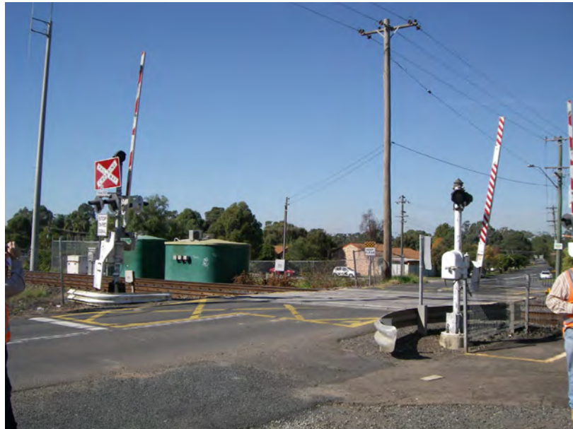
Fig. 6.20 Photograph of Camden Road Crossing
