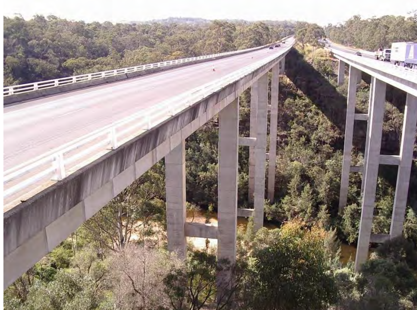
Fig. 6.23 Twin Bridges over the Nepean River at Douglas Park
