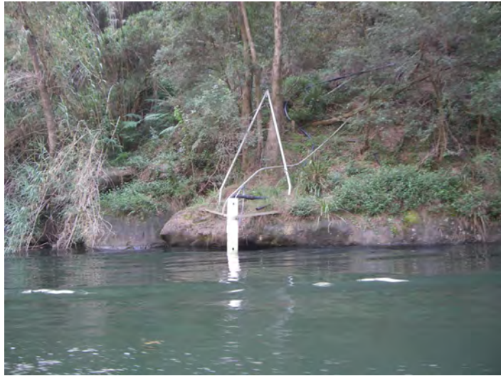
Fig. 5.17 Photograph of a Pump in the Nepean River
