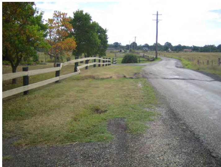
Fig. 4.10 Surface Compression Humping due to Low Angle Thrust Fault
