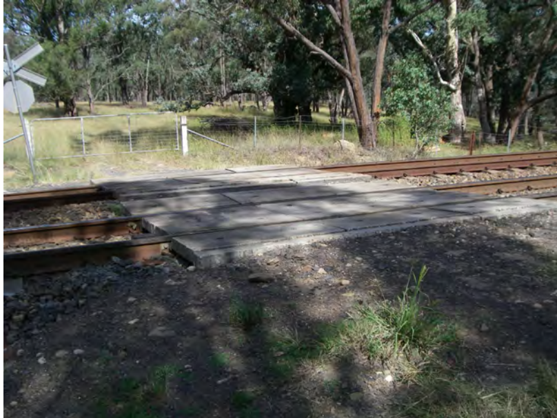
Fig. 6.21 Photograph of Vehicle Crossing at 76.13 km
