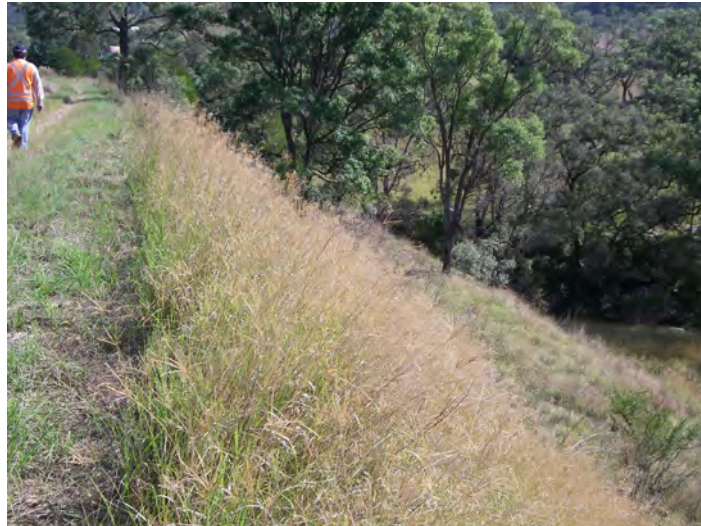
Fig. 6.17 Photograph of Embankment 75.7 km - Looking West (Down Track)
