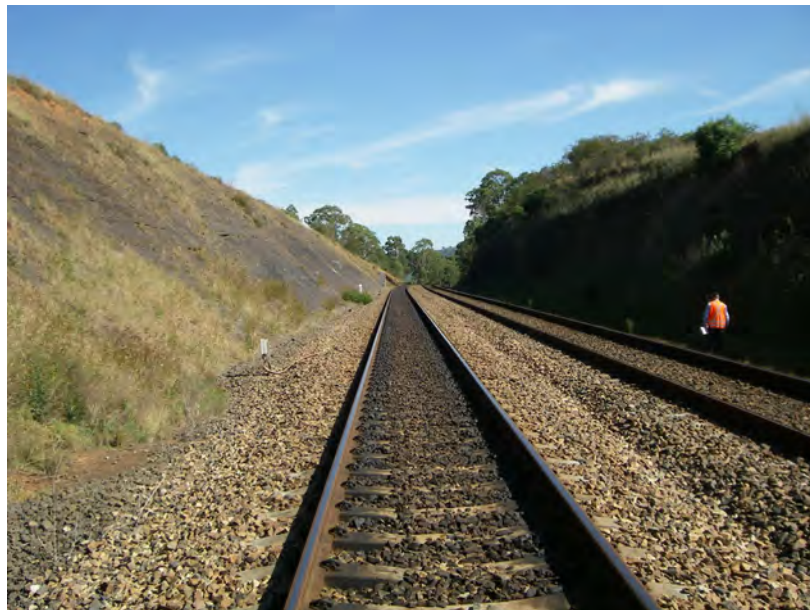
Fig. 6.12 Photograph of Cutting 76.6 km – Looking West (Down Track)
