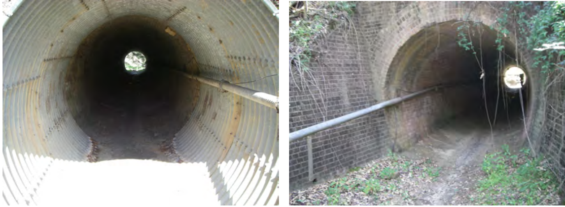
Fig. 6.5 Photographs of Railway Culvert at 76.212 km
