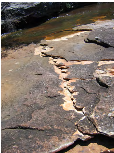
Fig. 4.15 Fracturing and Bedding Plane Slippage in Sandstone Bedrock in the Base of a Stream
