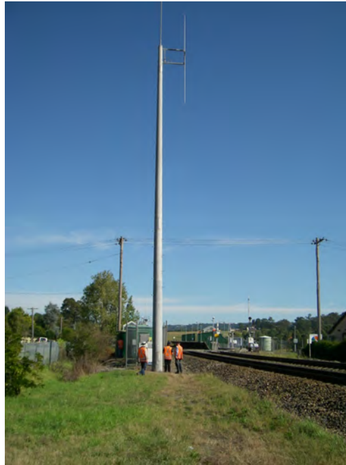
Fig. 6.22 Photograph of Communications Tower near Camden Road Level Crossing
