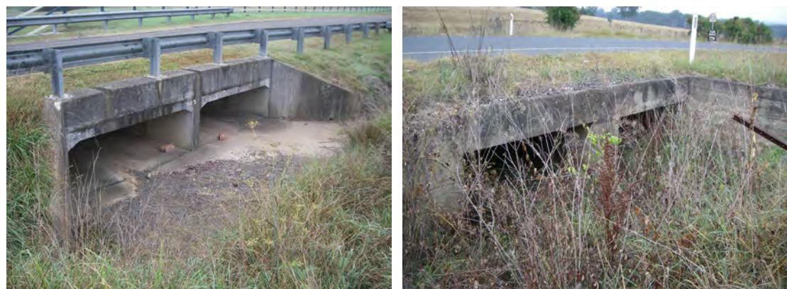
Fig. 6.35 Photographs of Box Culverts MR-A9-C07 (Left) and WW-C01 (Right)
