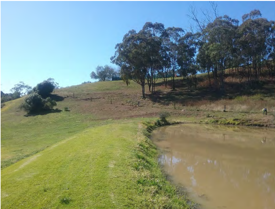
Photo 7 East facing photo showing disturbances from dam construction
