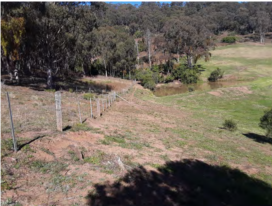
Photo 6 North facing photo showing disturbances from the construction of dams
