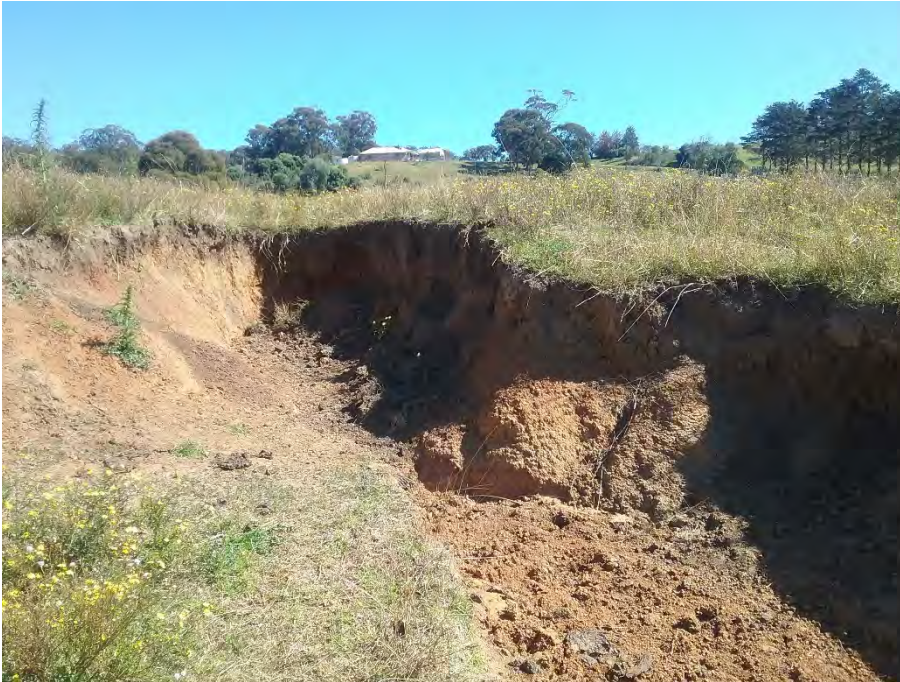
Photo 3 West facing photo showing exposure created by erosion
