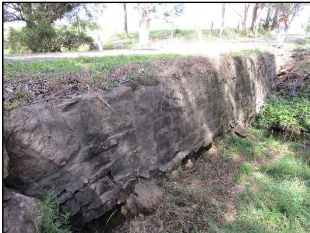
Plate 8: Stone culvert along Brooks Point Road, facing north east.
