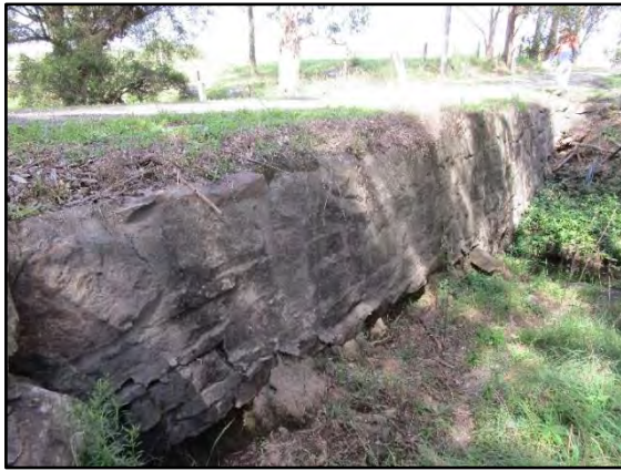
Plate 3: Stone culvert along Brooks Point Road, facing north east.
