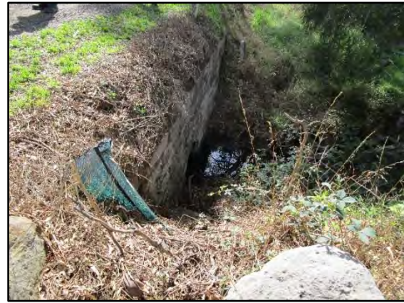
Plate 4: Stone culvert along Brooks Point Road, facing south west.
