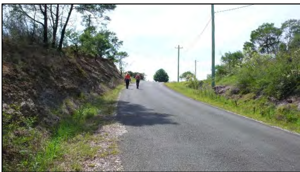
Plate 4: Example of high levels disturbance road cutting, construction and utility installation within the Subject Area.
