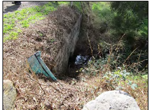
Plate 9: Stone culvert along Brooks Point Road, facing south west.
