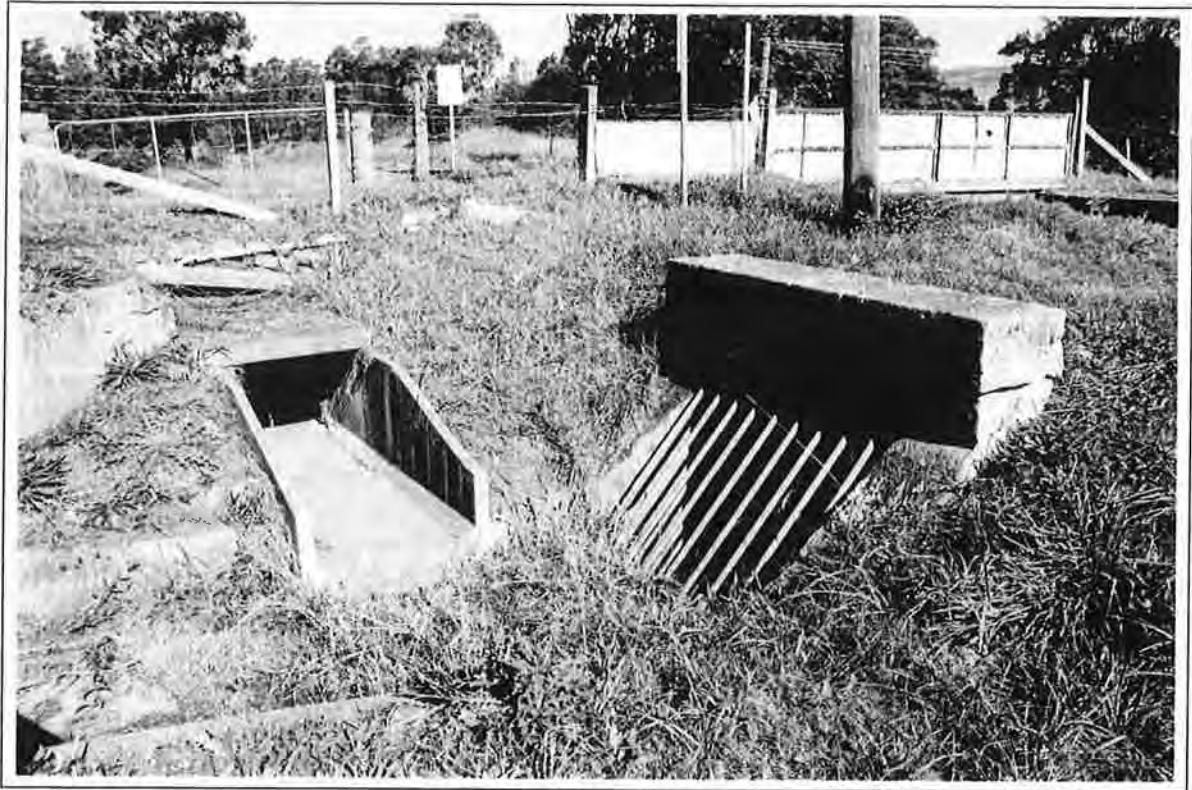
Caption Inverted syphon masonry culvert, Brooks Point Road
