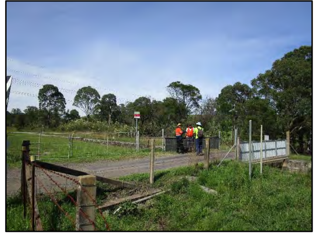
Plate 11: Canal overbridge at Brooks Point Road, looking south west.
