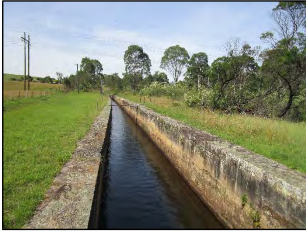
Plate 10: The Upper Canal, looking south from the canal overbridge on Brooks Point Road.
