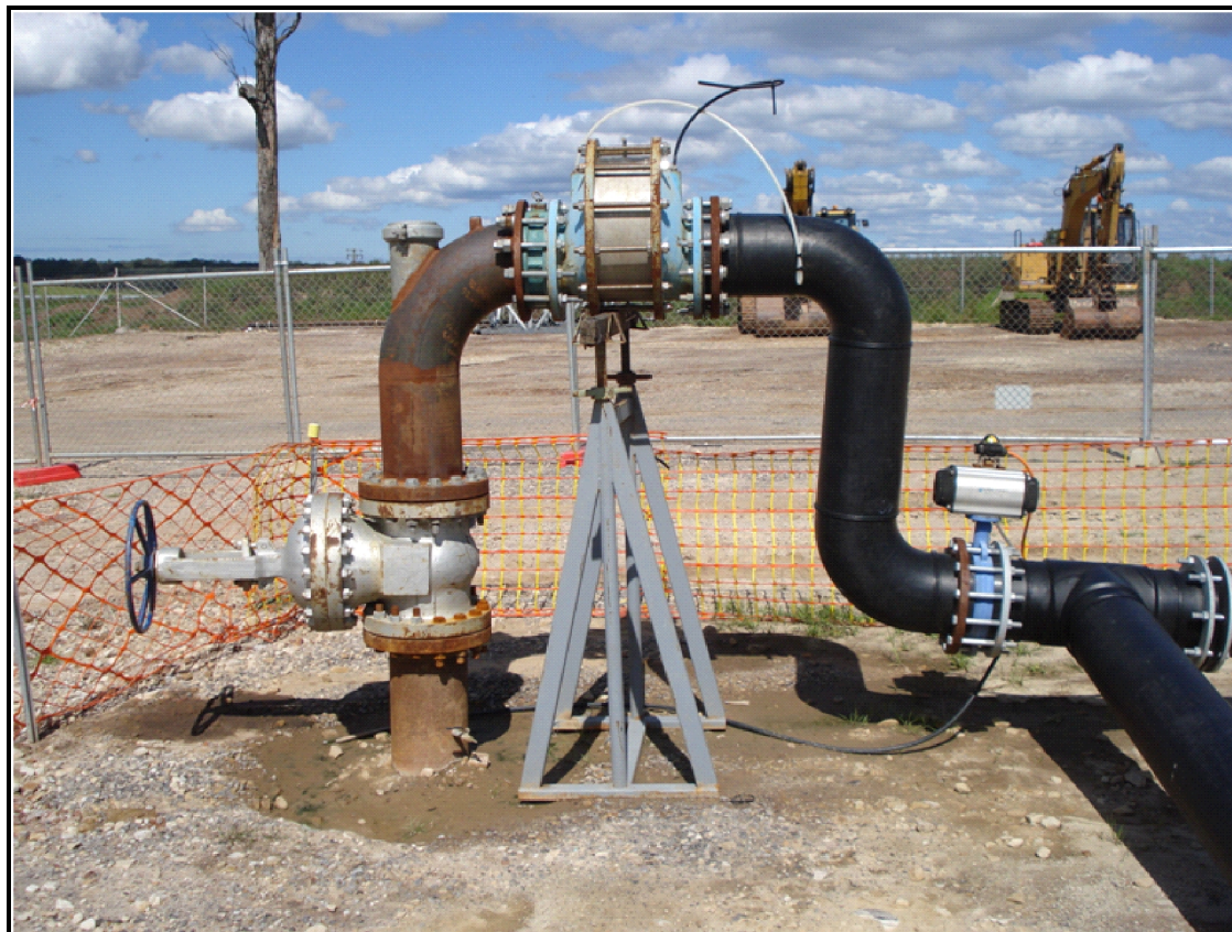
Figure 5.10 – Typical Wellhead Installation
