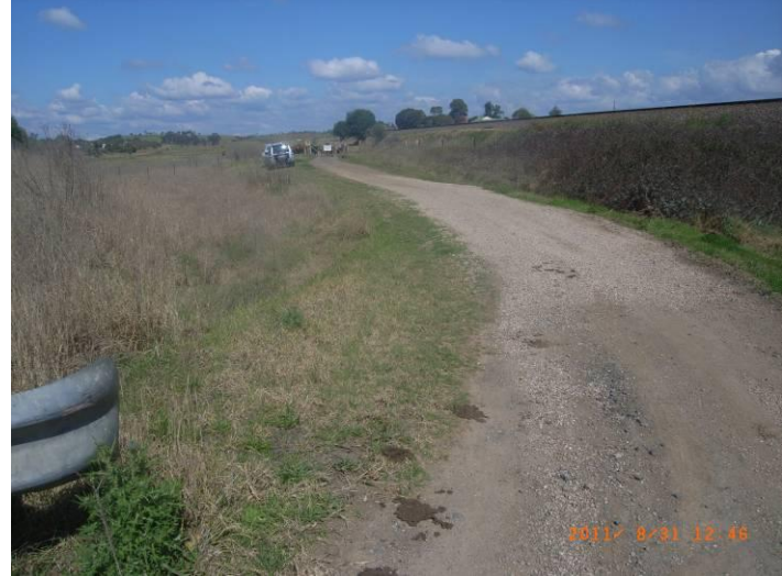
Photo 20 – Existing 705 MRD A/B access track off Morton Park Road
