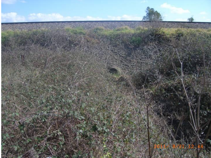
Photo 19 – 705 MRD A/B access requiring filling and drainage works
