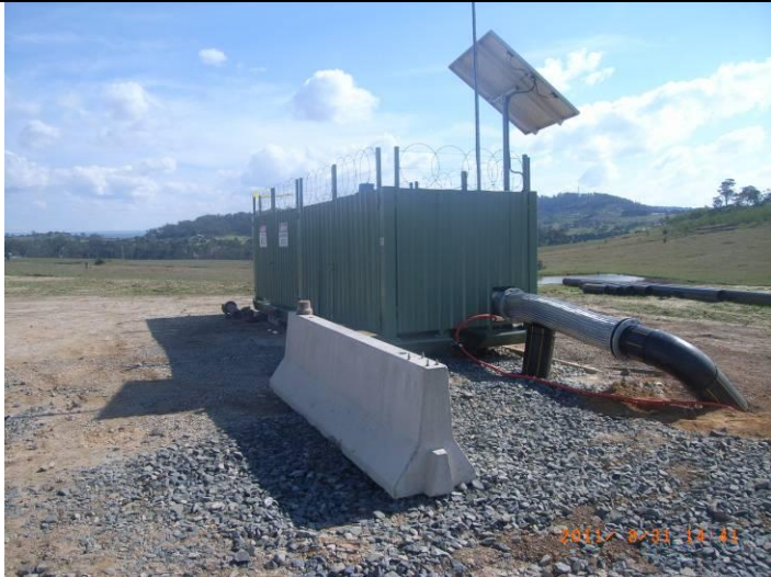
Photo 33 – Existing 704 MRD Site
