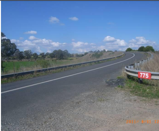
Photo 17 – LW705 MRD A B access of Morton Park Road looking east
