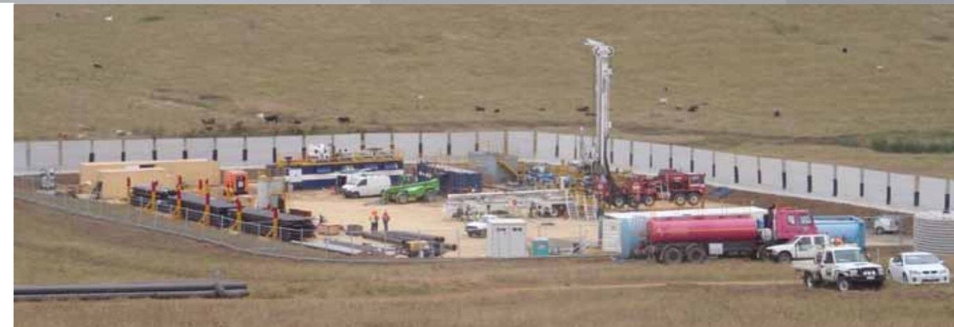
Illawarra Coal conducts mine safety gas drainage works in order to create a safe working environment underground. Once the surface gas drainage activities are complete the site is restored to its pre-work condition.
