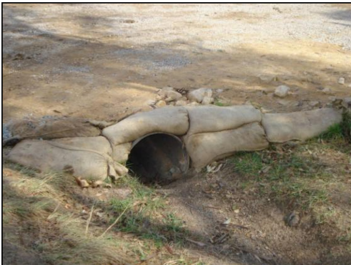
Figure 10 Erosion and Scour Control Structure
