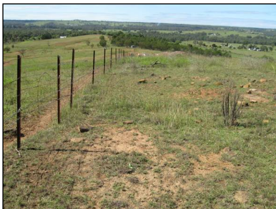
Plate 31: Location of Moreton Park Road IA-2 note the cut and fill scar on the western side of the fence
