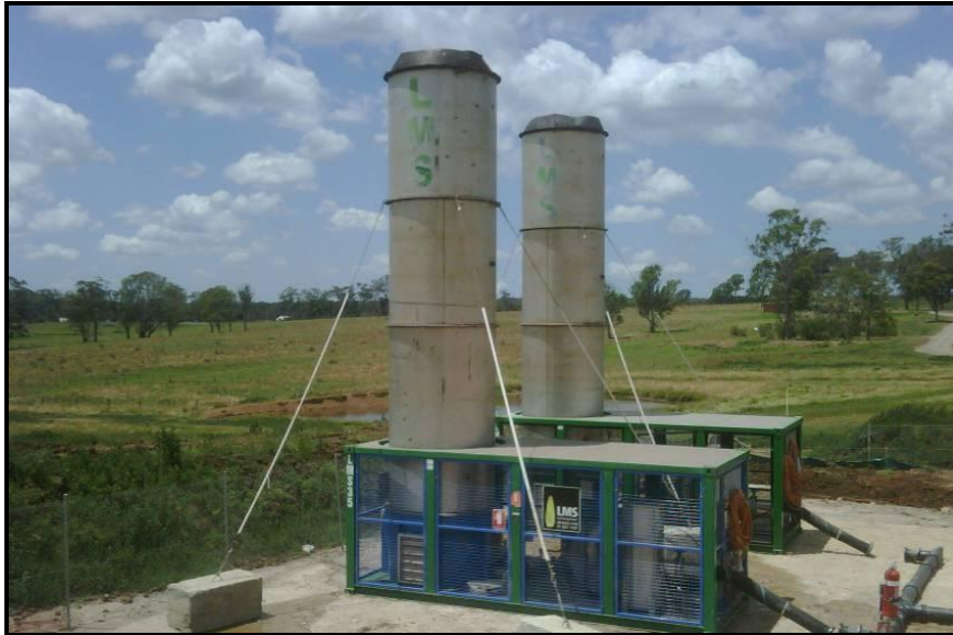
Figure 2.4 – Enclosed Goaf Gas Flaring Units
