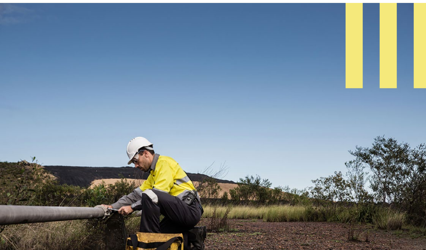
Inspecting our pipes at Illawarra Metallurgical Coal.
