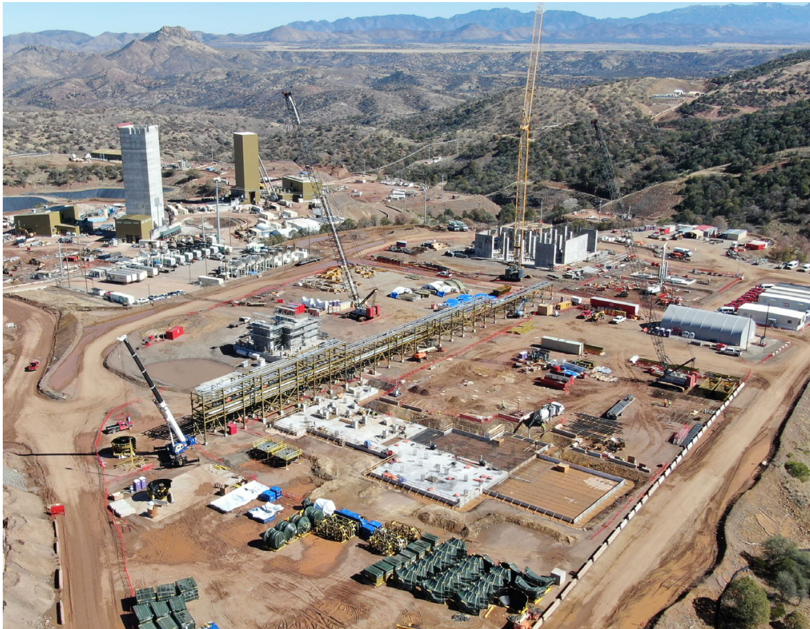
Surface infrastructure construction (January 2026)
